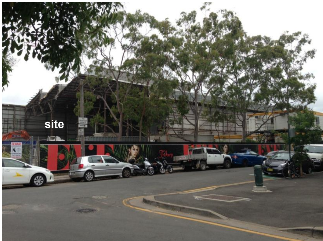
Figure 4: View of the subject site from Eve Street looking northeast
