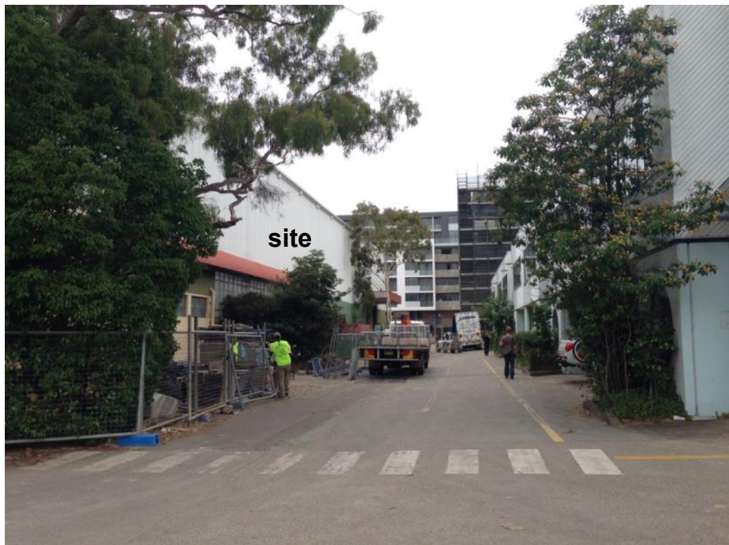
Figure 10: View of the subject site looking west along the existing ROW (future pedestrian through link) with the Erko development in the background
